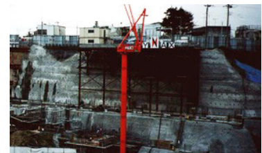
Temporary landslide prevention walls for condominium construction
