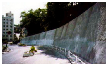
Reinforcement of existing retaining walls: shotcrete finish
