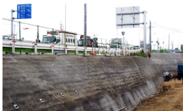
Temporary landslide prevention for a cut site in the widening of National Route 1 (construction case 4)
