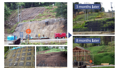
Ground reinforcement (part of construction case 3), tree planting finish
