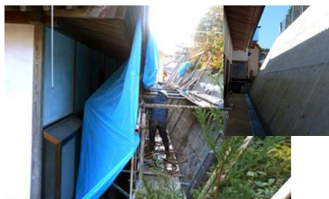
Reinforcement of existing retaining walls. Min. distance from residential areas: 1.7 m; manual drilling (construction case 1), concrete placement finish
