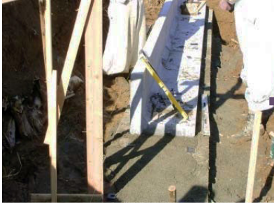
① Panel foundation construction
