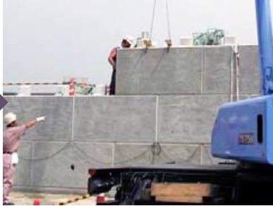
② Panel piling/connection
