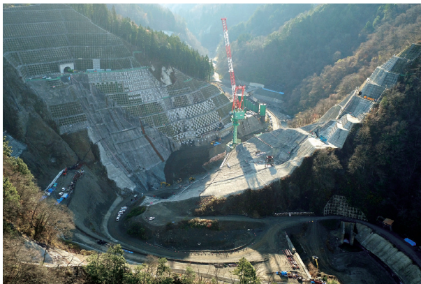
Uchigatani Dam construction (Gifu Prefecture)
