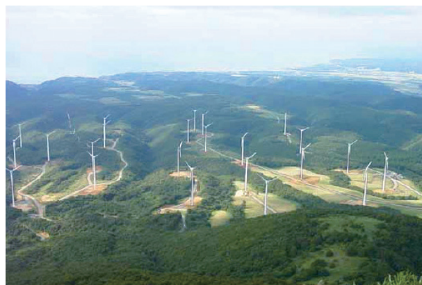
Esashi wind power generation project
