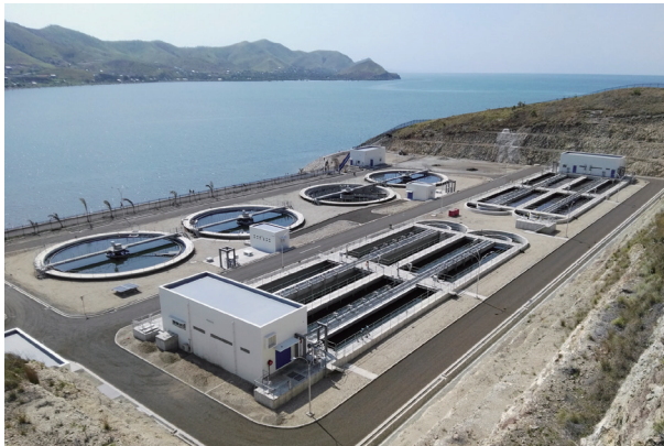
Joyce Bay sewage treatment plant, Port Moresby
