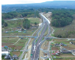
Improvement of the Sakuho Section of the Chubu Odan Expressway (6) (Nagano Prefecture)
