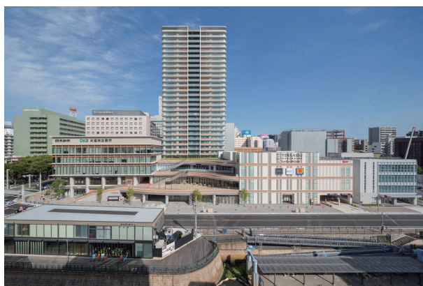
Terrace Nayabashi (Prime urban redevelopment for the Nayabashi eastern section)
