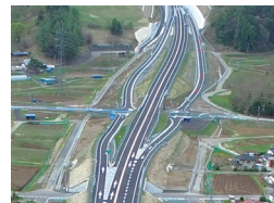
Road made with recycled gravel
