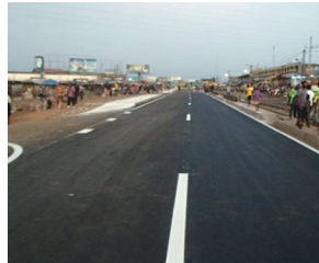
Project for Reconstruction of Somalia Drive in Monrovia (Republic of Liberia)
